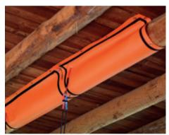
SAMITECH is revolutionising the pest control sector by improving classic heat treatments with a new technology based on far infrared waves that penetrate deep into the objects surface killing insects by dehydration.
